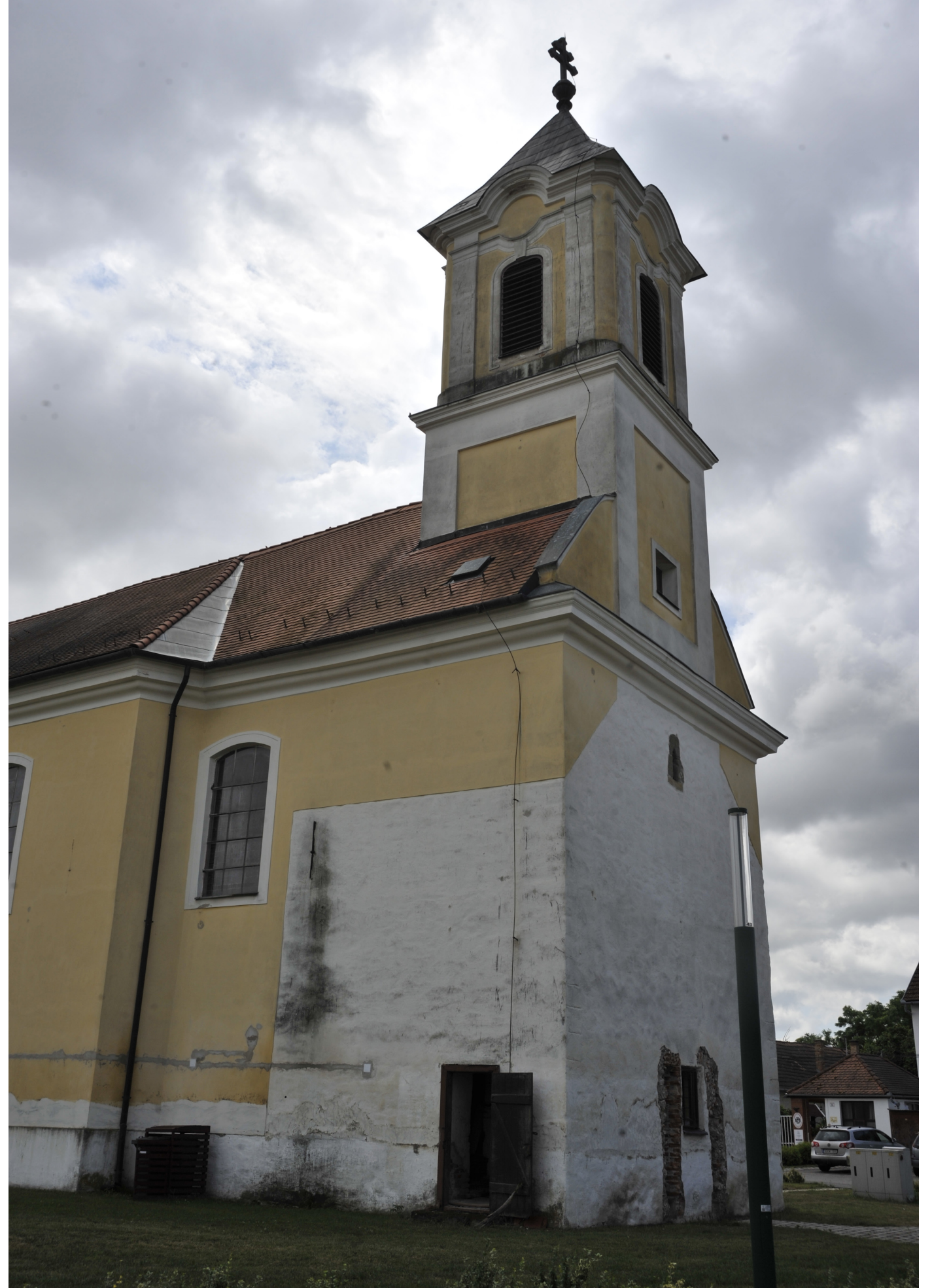
51/1 Templomtorony / Church tower
