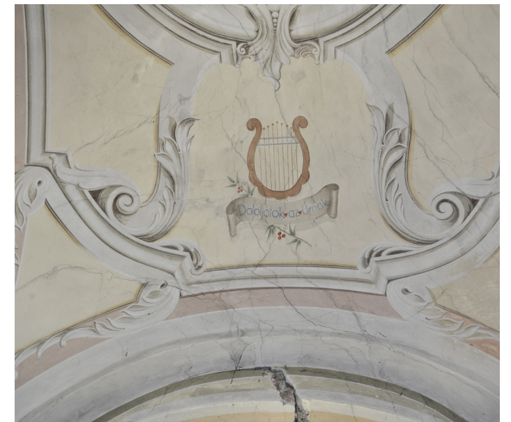
59/3 Festés állapota, kipergés / The condition of the paintings, flaking
