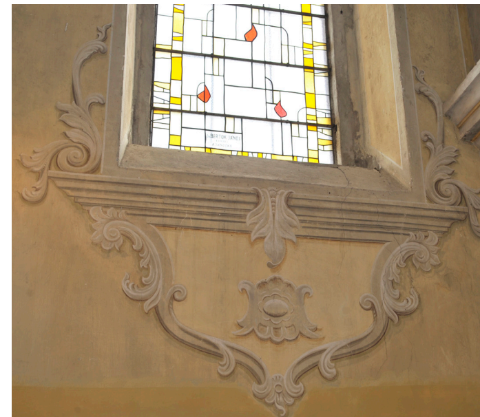
59/2 Ablak alatti festett ornamentika / Painted ornaments beneath the window
