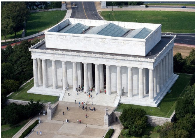
FIGURE 17 AERIAL VIEW OF LINCOLN MEMORIAL: CAROL M. HIGHSMITH
