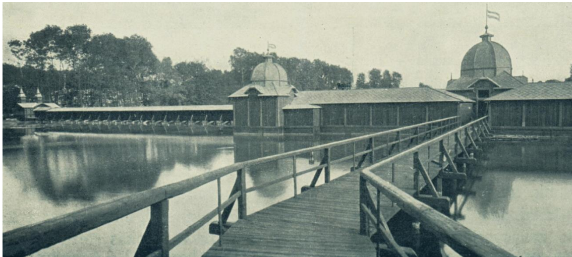
Figure 68 Covered and open bridge connected to main building and the entrance.
