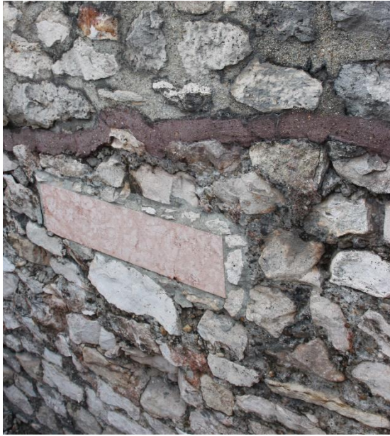
Figure 9 Stone wall structure with marble plaque
