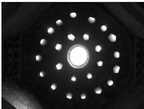
Figure 17 The configuration of light openings on the central (a) & on one of the peripheral domes (b) of the hot chambers in Bey Hammam
