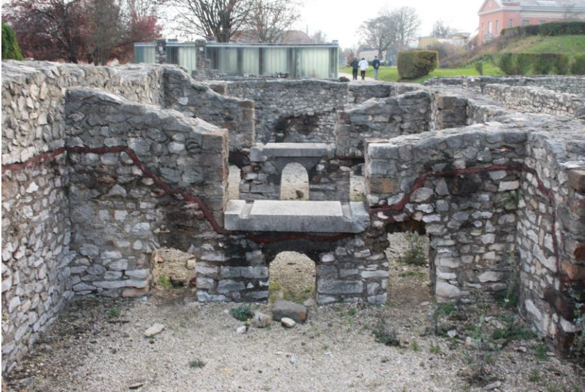
Figure 7 Arched openings of the hypocaust system
